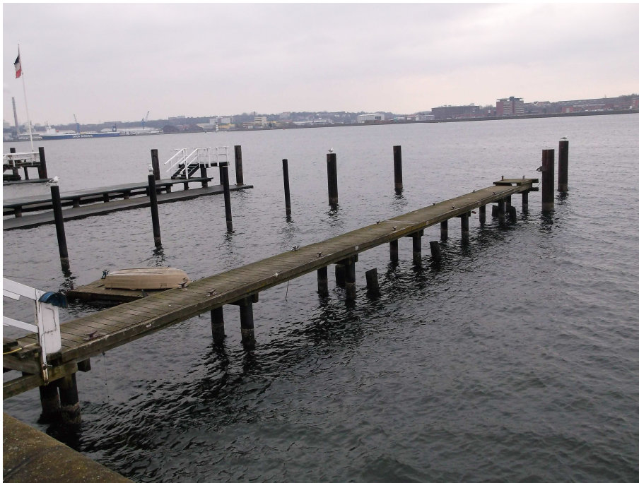
Figure 2.3 Wooden bridge with berths typical in Kiel Fjord region (Source: GuntramSeiß).
