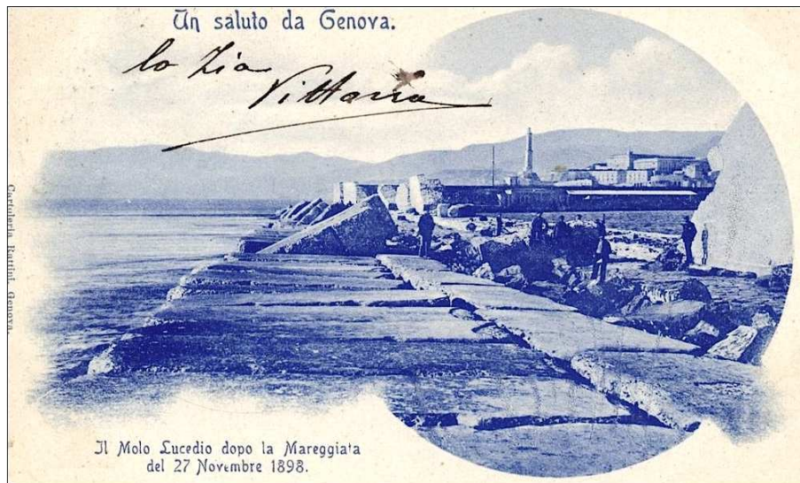
Figure 7.16 Photography of the Lucedio dike (Genoa) damaged by storm of November, 1898 (Source: unknown).
