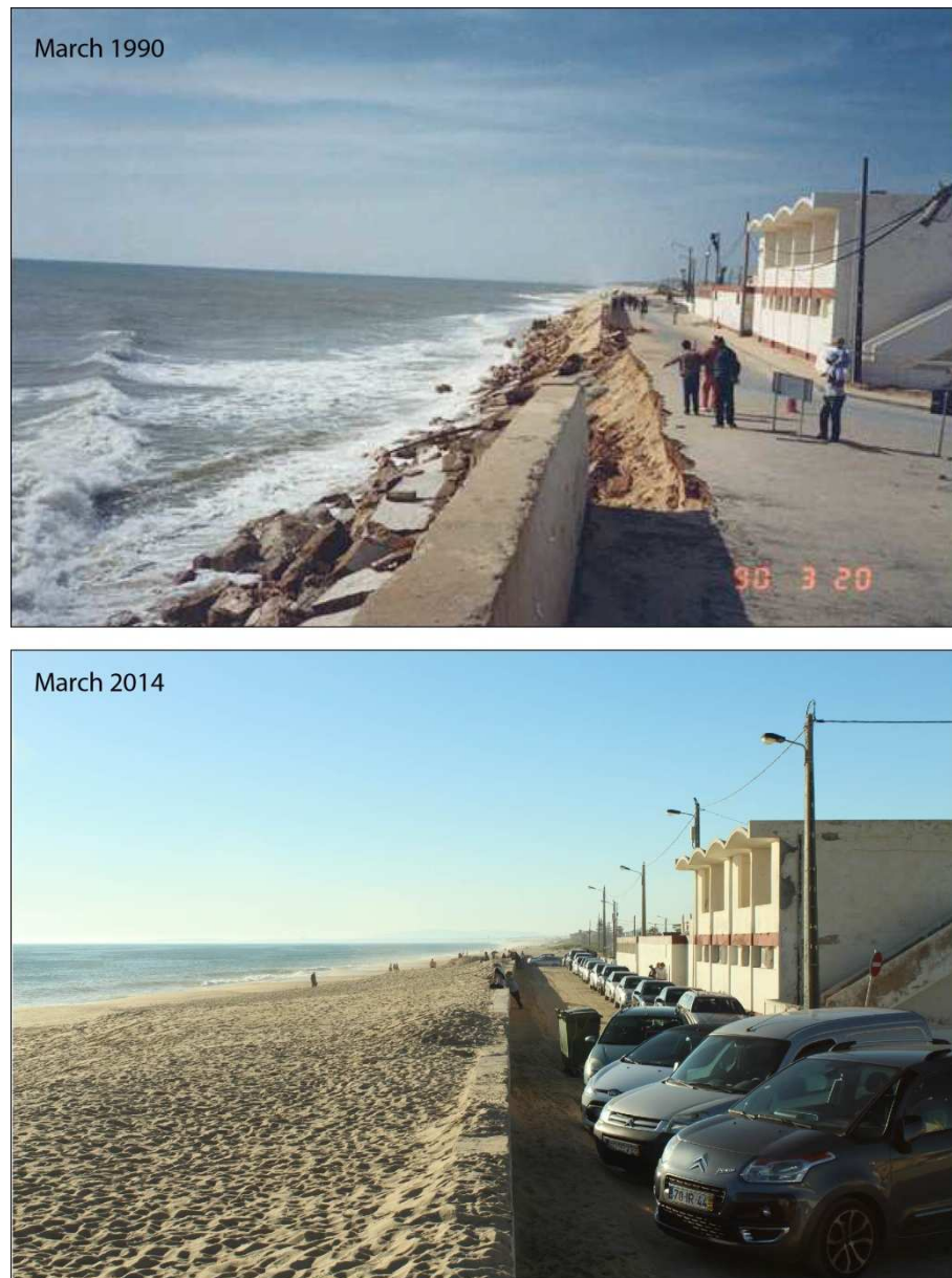
Figure 7.10 Praia de Faro after the 1990 storm where the road was damaged and presently.
