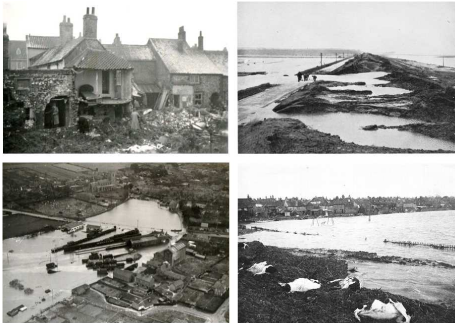
Figure 7.4 Wells immediately after the 1953 storm surge. Top left: Houses on Freeman Street, showing how the back walls had been destroyed by the surge. Top right: Large breach in the Great Wall on the western side of Wells Harbour. Bottom left: The railway station and tracks completely flooded. Bottom right: Dead livestock and other debris left from the surge. Photos provided by John Tuck, except top right from Steers, 1953.
