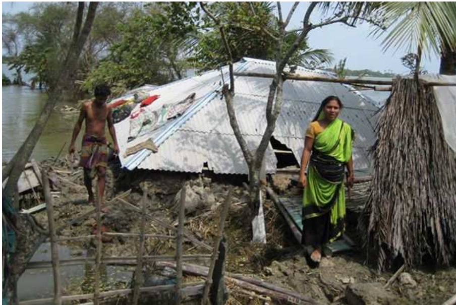
Figure 2.11 Damaged home and the affected homeowner, after the occurrence of an extreme event in Sandwip Island (Source: risckit.eu).
